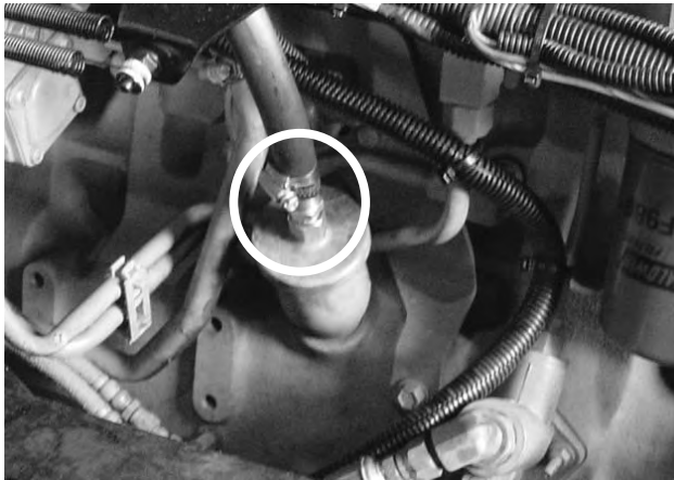
Example 2: Check-valve adapter welded onto fill tube
