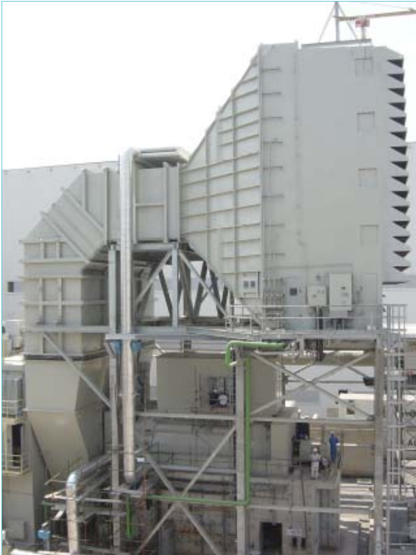
Above: The inlet bleed heater
