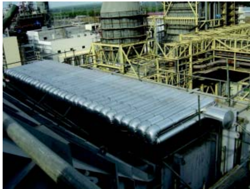
Above: The inlet bleed heater
