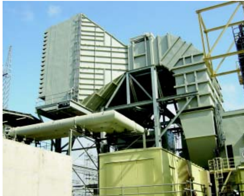
Above: The inlet bleed heater
