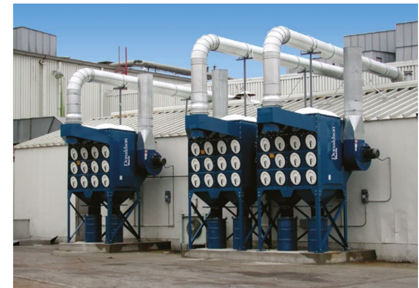
DFO on Metalising Powder Flame 34,822 m 3 /h (20,500 cfm)
