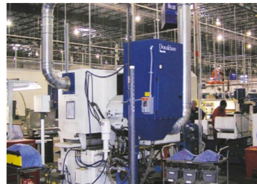
WSO at M3 Achining Centre 2,038 m³/h (1,200 cfm)
