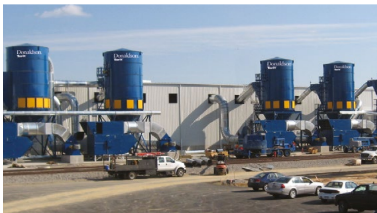
RF - Wood Furniture Facility 684,556 m 3 /h (403,000 cfm)
