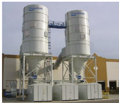
LP on Wood Dust 271,784 m 3 /h (160,000 cfm)
