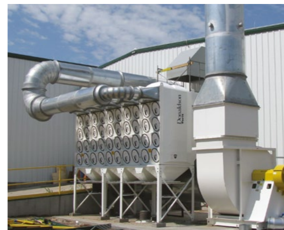
DFO on Corn Husking & Sorting 48,412 m 3 /h (28,500 cfm)
