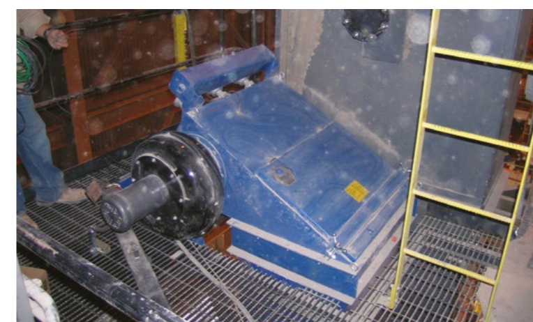
CPV - Bucket Elevator 2,038 m 3 /h (1,200 cfm)
