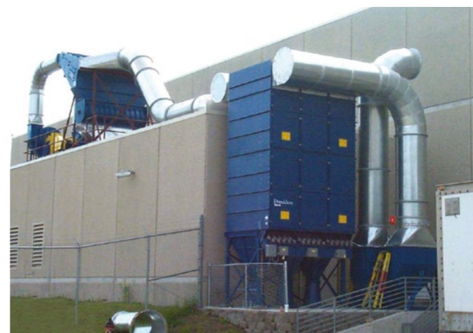
DLMC on Paper Dust 45,864 m³/h (27,000 cfm)
