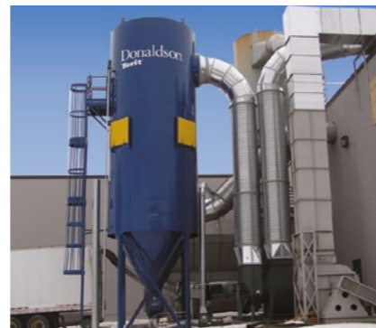
RF - Cabinet Shop 82,385 m 3 /h (48,500 cfm)
