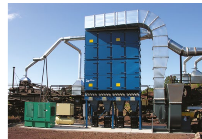
DLMC on Rock Crushing 69,645 m³/h (41,000 cfm)
