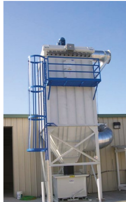
FS on Woodworking 33,973 m 3 /h (20,000 cfm)
