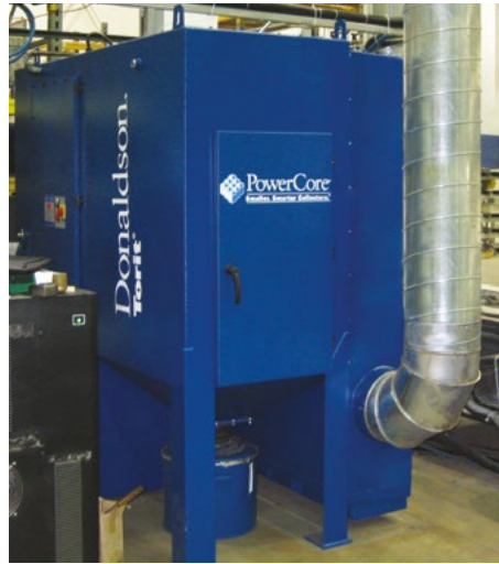
TG on Plasma Cutting 3,900 m 3 /h (2,300 cfm)
