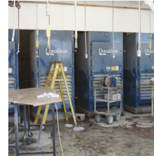
DWS on Granite Finishing 37,370 m³/h (22,000 cfm)
