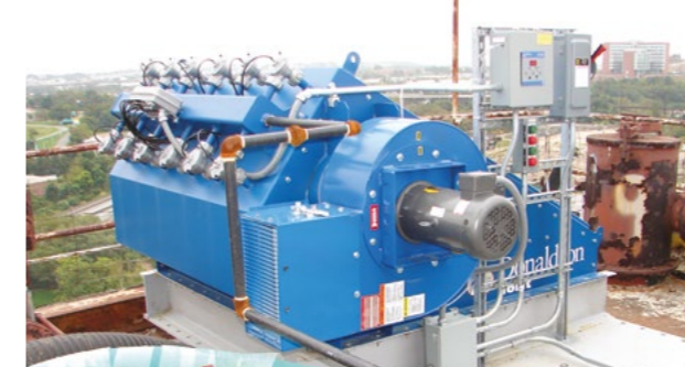
CPV - Multiple Cement Silos 8,154 m 3 /h (4,800 cfm)
