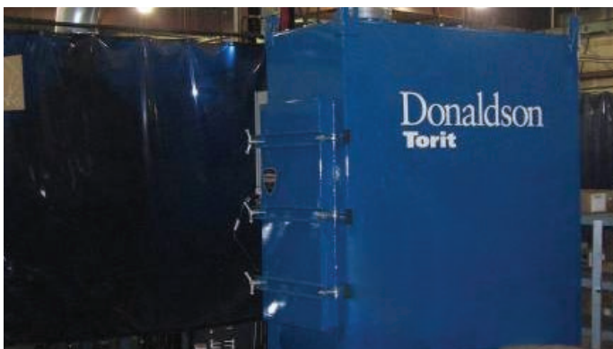
TG4 on Welding
