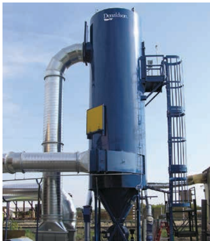
RF Dust Collector
