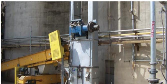
Installed on the boot section **1** and discharge point **2** of the elevator, PowerCore® CPV eliminates the need for costly ducting.
